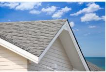
ASPHALT SHINGLES Three-year weathered SRI range: 14-34
