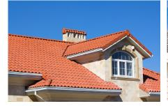
TILE (CLAY & CONCRETE) Three-year weathered SRI range: 4-91
